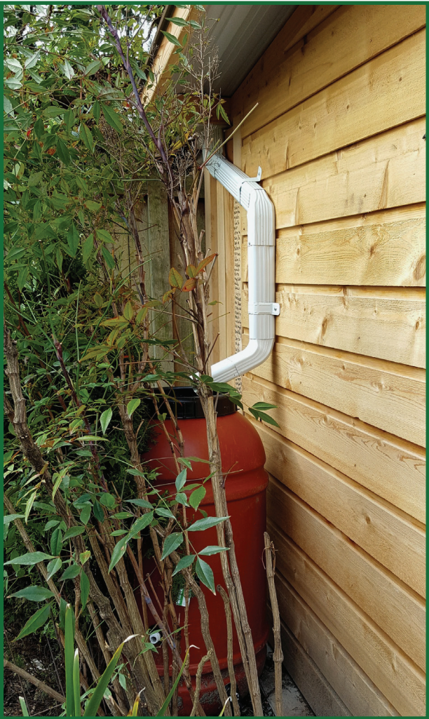
Jackson Park P-Patch's renovated shed features handicapped-accessible doors and concrete flooring, with permeable paving surrounding it. A partially hidden cistern (below) collects rain water from the shed roof.
