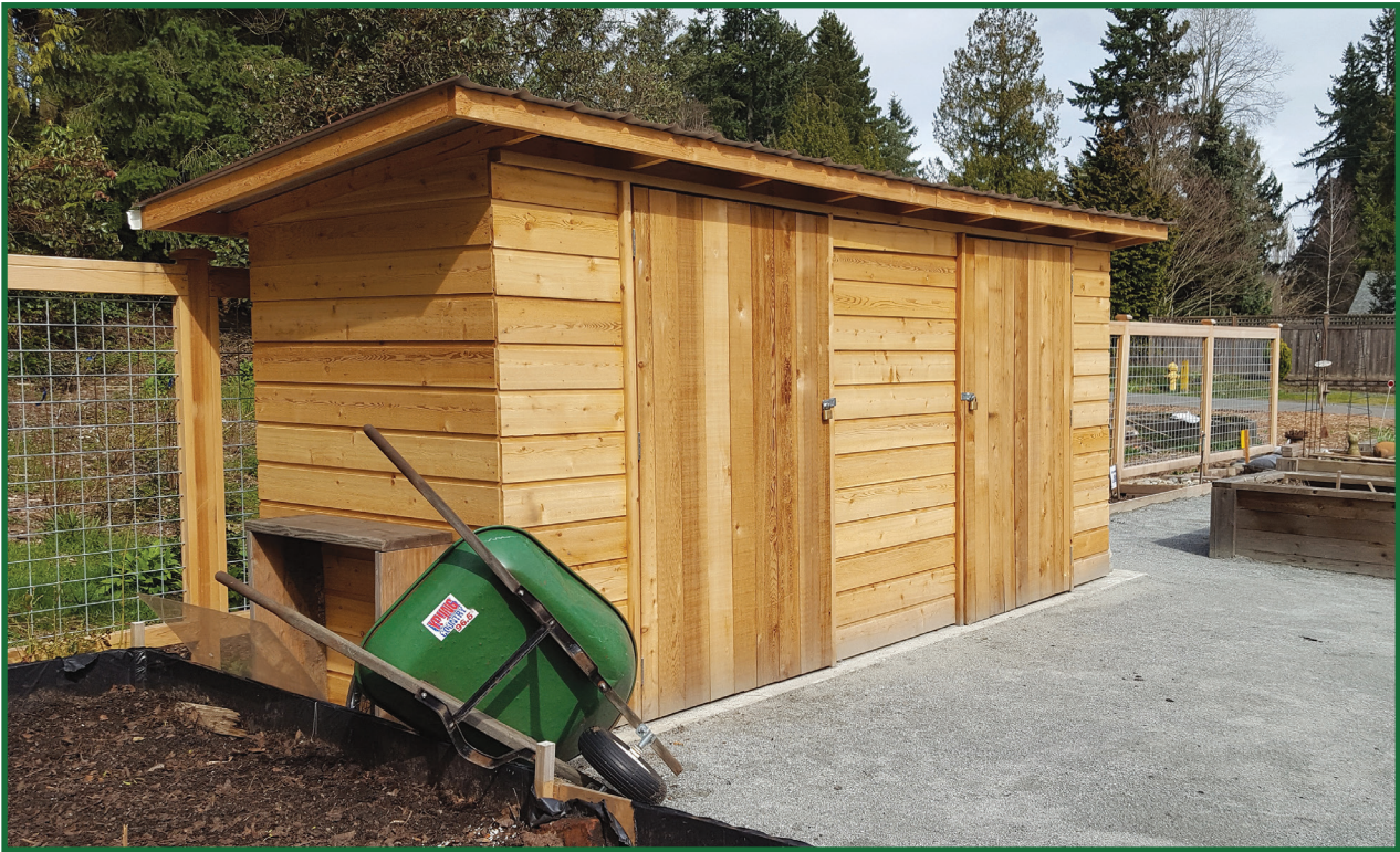
Jackson Park P-Patch's renovated shed features handicapped-accessible doors and concrete flooring, with permeable paving surrounding it. A partially hidden cistern (below) collects rain water from the shed roof.
